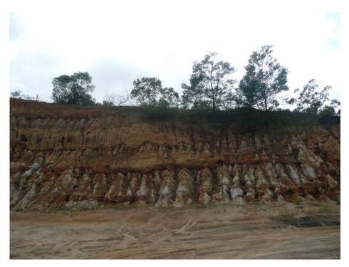
Figure 5: Area of erosion within Glenfield Waste Facility
